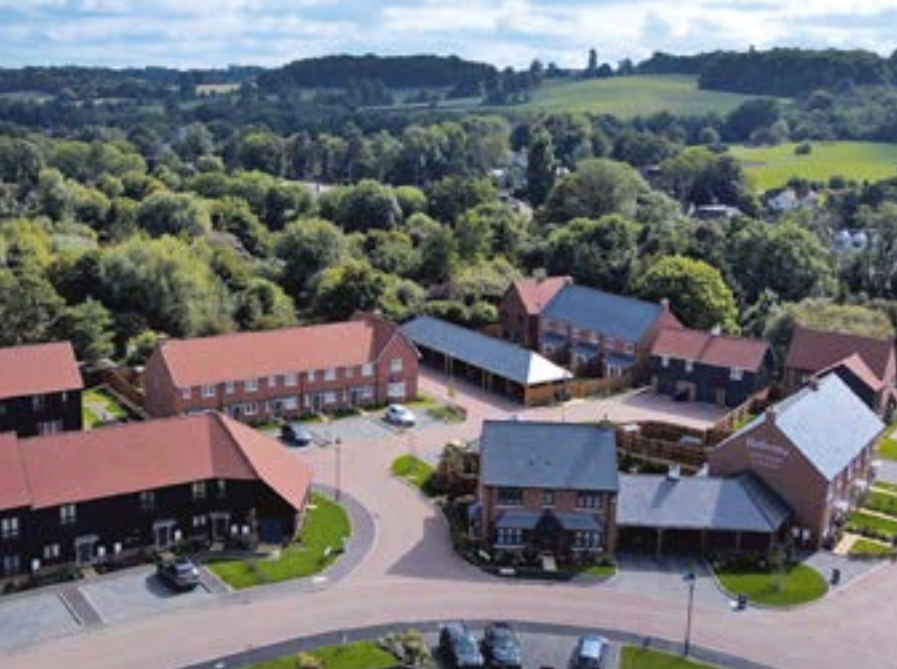
← Aerial view of our Westbrook Moorings development in Hertfordshire.
